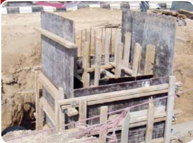
Sewage / Rainwater Drainage Works
